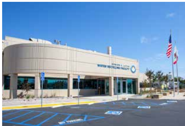
The Edward C. Little Water Recycling Facility has produced more than 200 billion gallons of recycled water.
