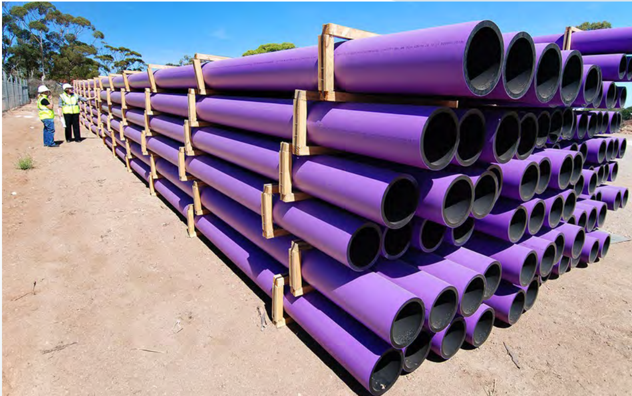
Recycled Water Pipes
