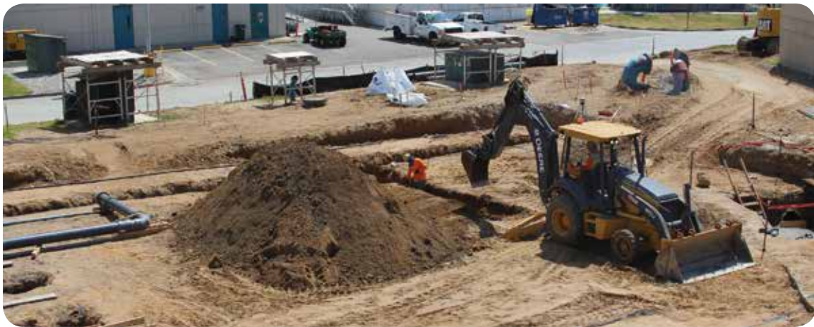
Edward C. Little Water Recycling Facility Construction
