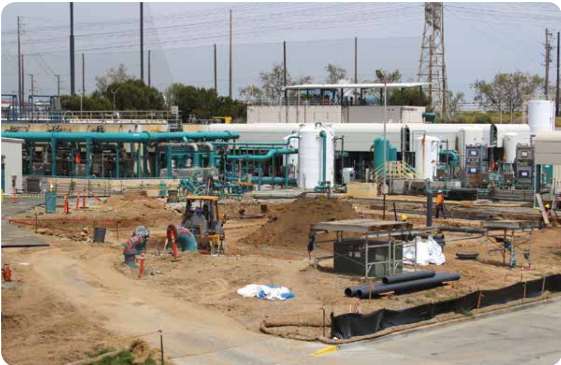
Edward C. Little Water Recycling Facility Construction
