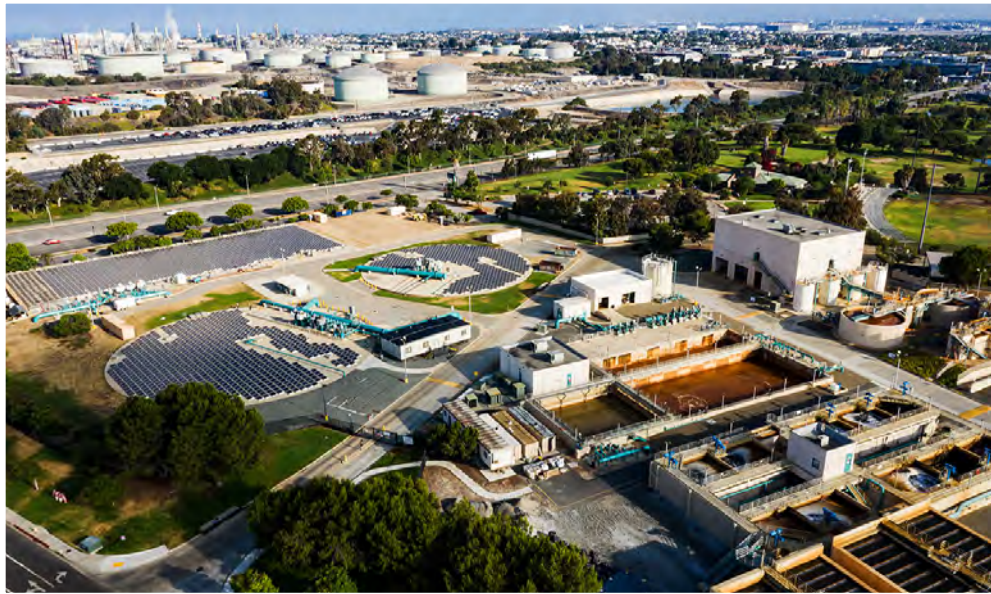
The western side of ECLWRF, with the product pumps, Title 22 filters, and dewatering building shown
