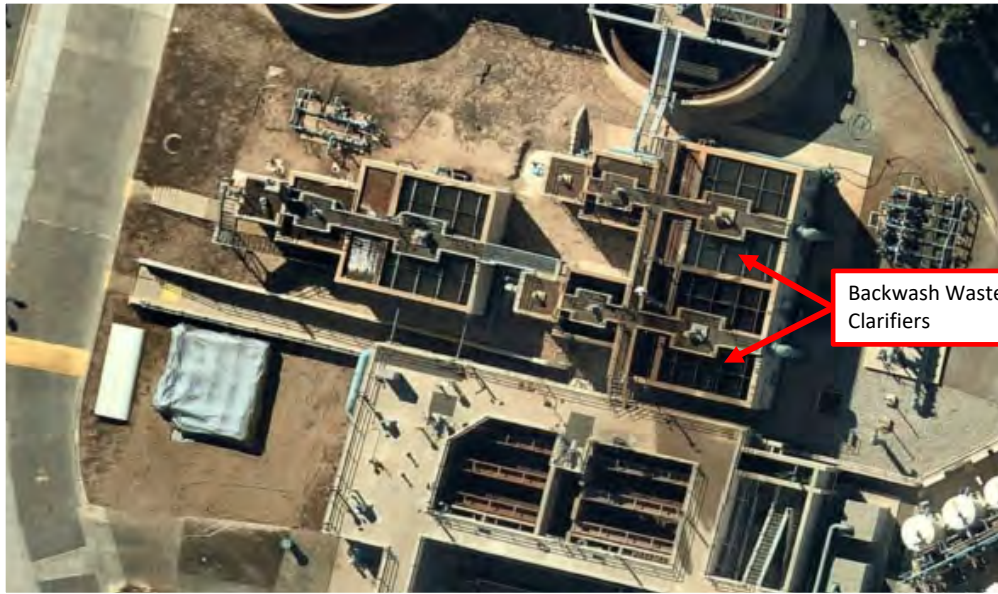
Backwash Waste Clarifiers at ECLWRF
