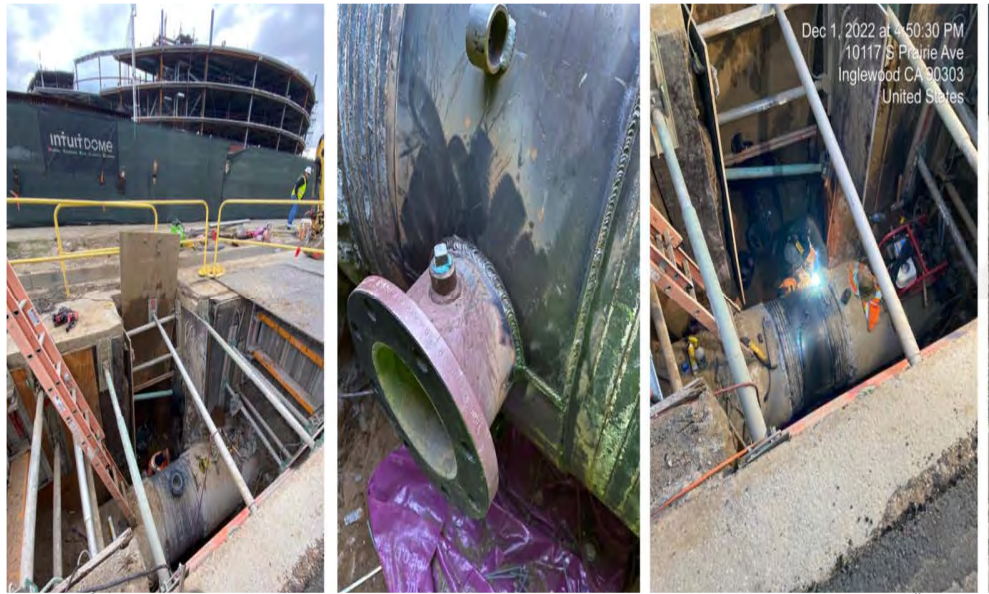
Left photo to Right photo: Project Site, 6-inch welded Nozzle outlet, Welded Wrapper Plate onto 36" existing pipeline
