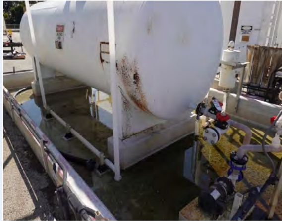
Left Photo: Sulfuric acid bulk storage tank. Right Photo: Sulfuric acid carrier pipe.
