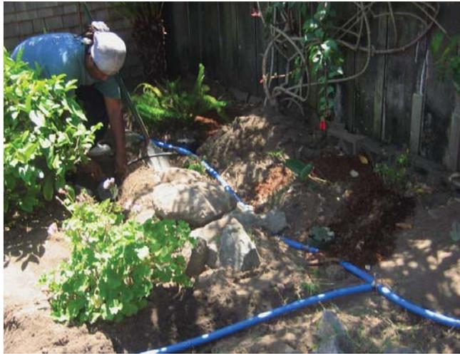
*1-inch Blu-lock HDPE tubing laid out in trenches. All tubing was buried after system was finished.
