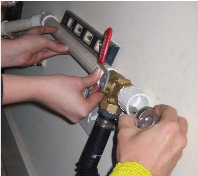
*Gluing pipes on either side of a 3-way valve.
