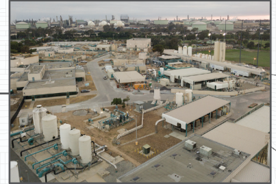
Edward C. Little Water Recycling Facility
