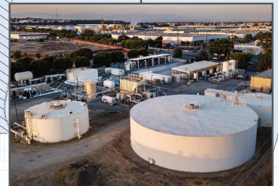
Juanita Millender-McDonald Carson Regional Water Recycling Plant
