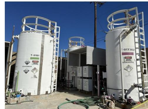
2,375-gal sodium bisulfite tanks at CNTP
