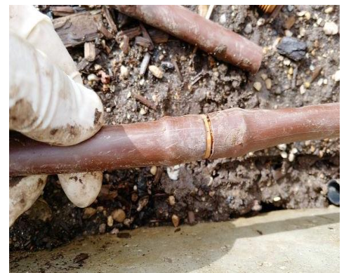
Insert Coupling and Reattach
